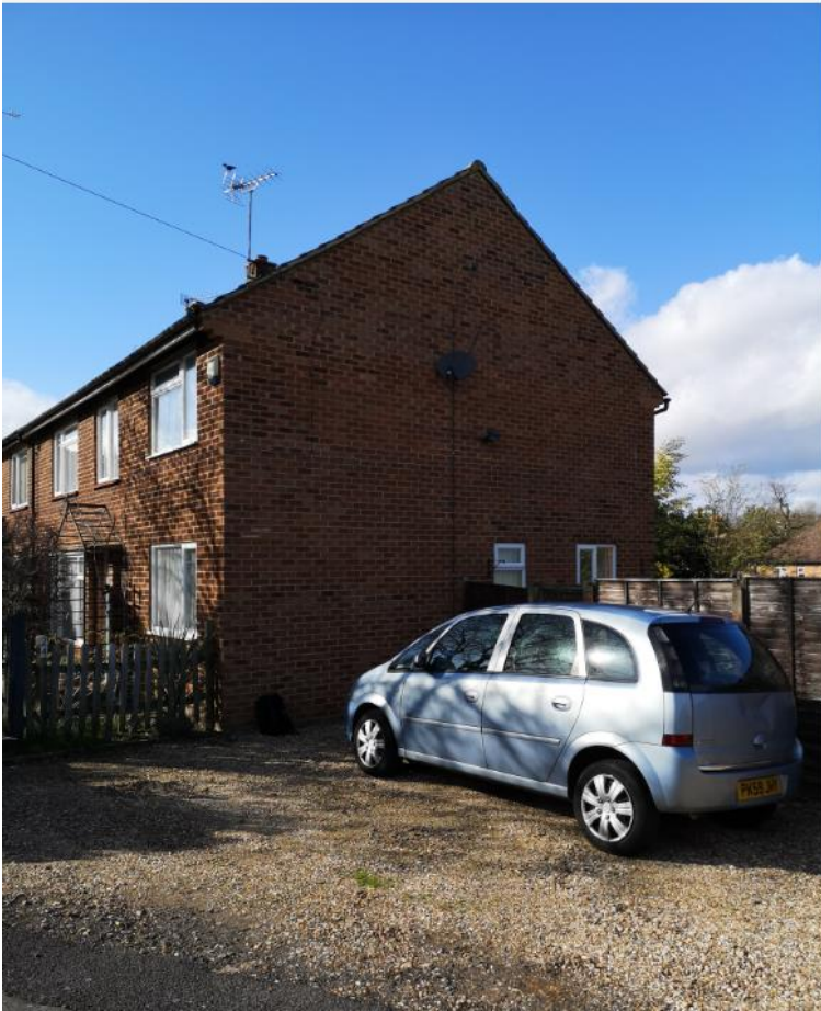
Existing site photos Front / side
