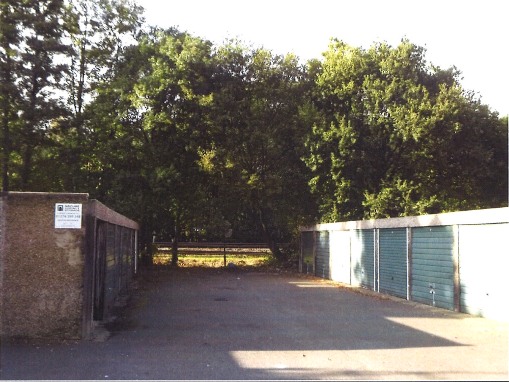
Garage Block and railway beyond
